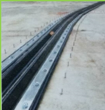
Waterstop before placement of cover 覆盖之前的止水带
